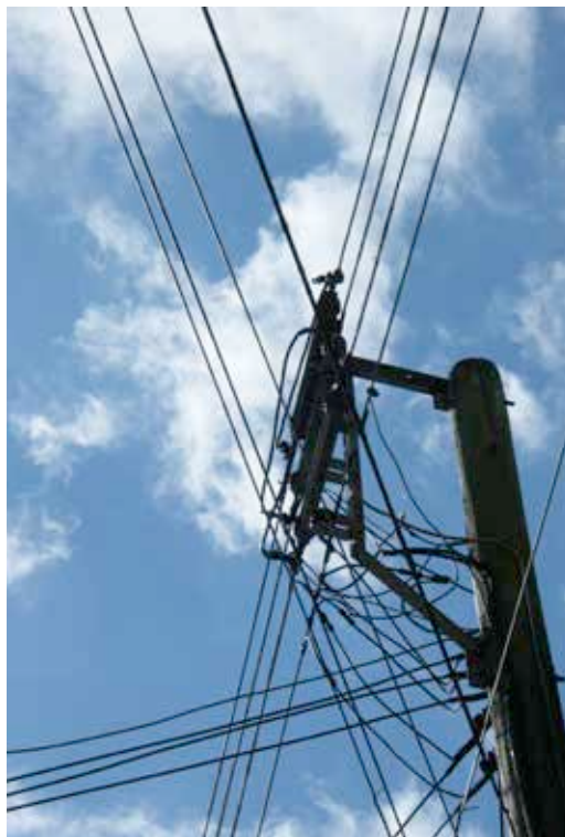
Overhead power and telephone cables are considered by many to be intrusive and unappealing. © Tristan Dewhurst
